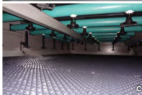
D. Phoenix cooling towers utilize CCS's patented 2- and 3-bolt connection system, creating a stronger connection and a more stable structure.
